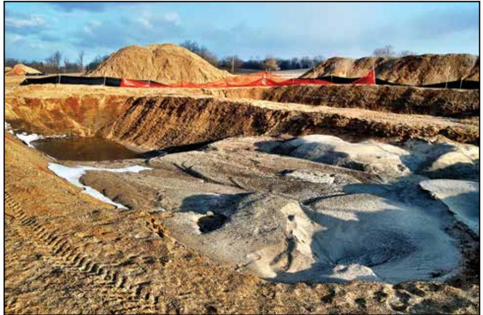
**The material removed using the Sand Wand™ is pumped to discharge or dewatering pits. These pits are temporary and excavated in upland areas.**
